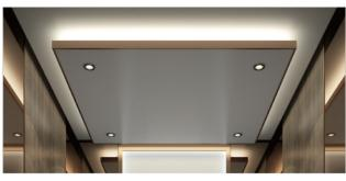
Lighting: ambient floodlight lighting, central down light direct lighting Material: central painted steel plate, Titanium-coated hairline stainless steel frame two-side painted steel plate Thickness: 200mm
