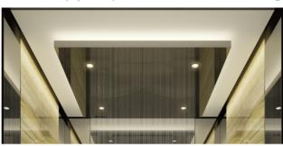
Lighting: ambient floodlight lighting, central down light direct lighting Material: central mirror stainless steel, ambient Painted steel plate Thickness: 200mm
